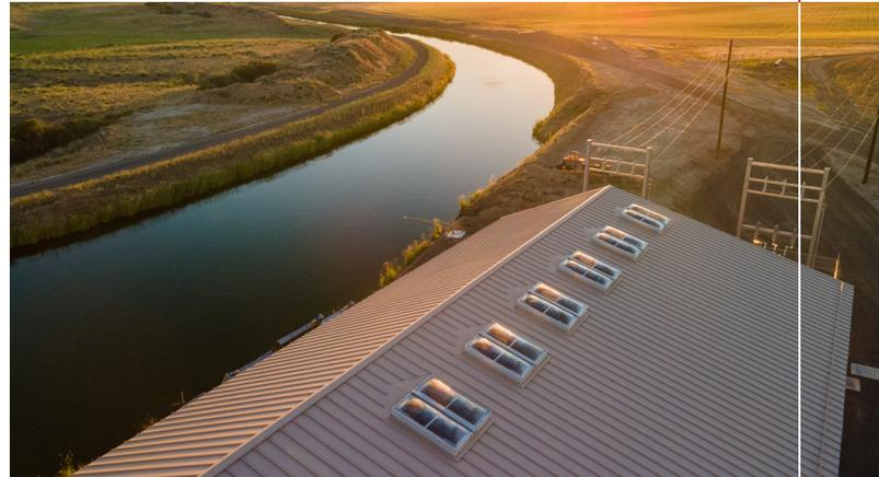
Teams will access the pumps through roof hatches manufactured by The BILCO Company. The custom hatches are fabricated with polycarbonate dome covers for natural daylight and engineered lift assistance for easy, one-hand operation. They are also modified for hand winch operation, allowing them to be easily opened and closed from inside the building.
