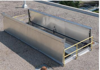
lift and lower the centrifuges into the building through a custom sized roof hatch manufactured by BILCO. The large roof hatch was equipped with engineered lift assistance to afford safe, and easy one-hand operation and will allow the centrifuge to be easily removed if it ever needs to be repaired or replaced.
